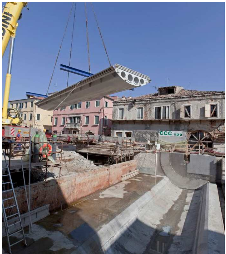
5. At work installing the Santa Maria floodgate in Chioggia.
