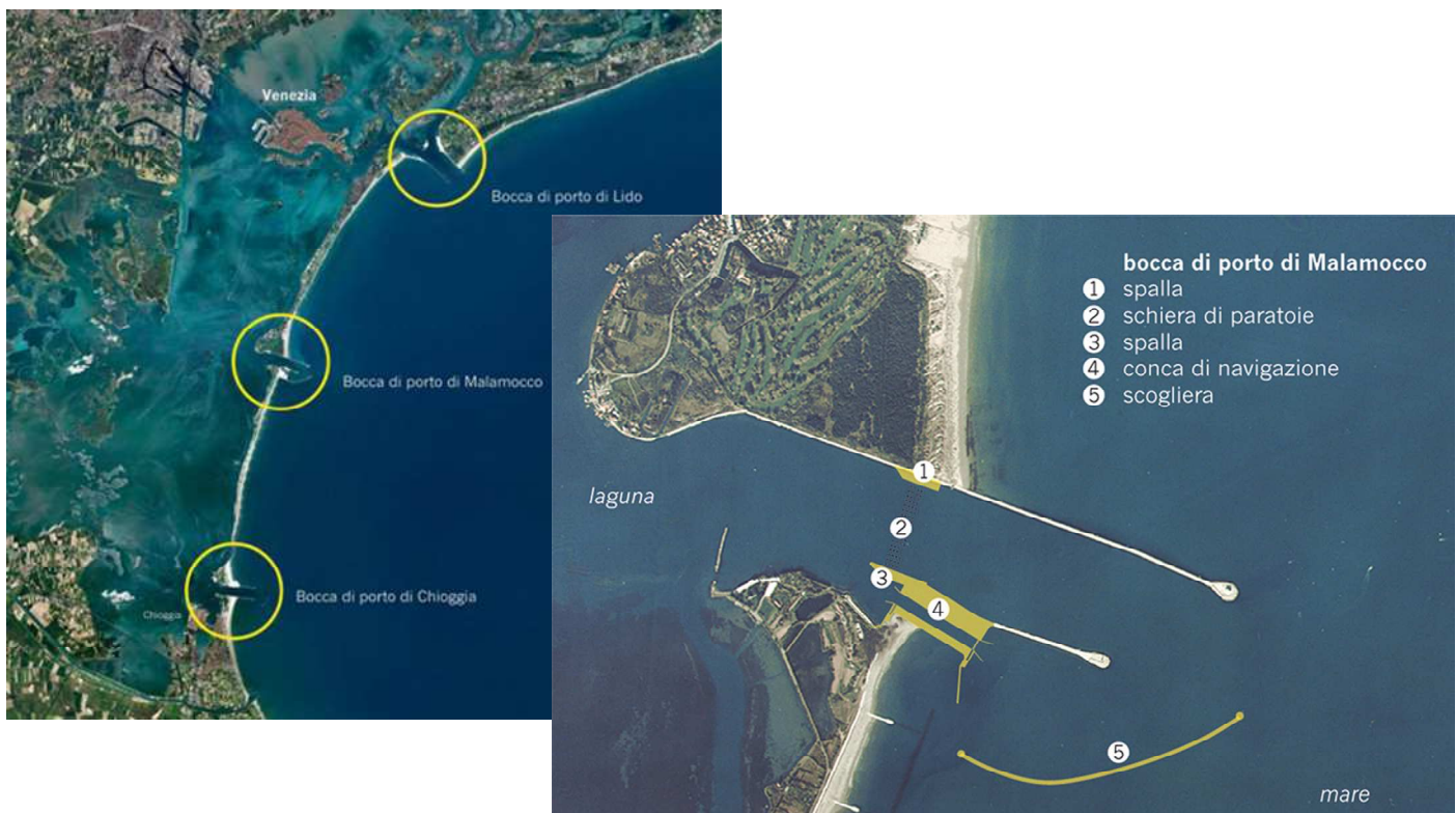
1. Venice inlet with threshold and shoulder caissons
