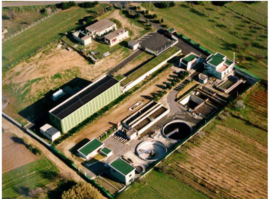
The wastewater recycling and purification plant in Villasimius (CA).
